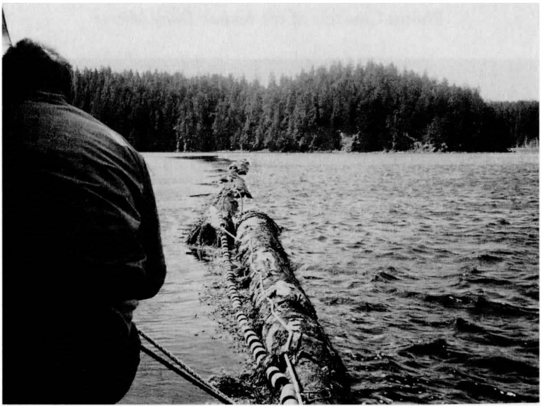
Makeshift booms were deployed in hopes of keeping oil out of sensitive bays.
